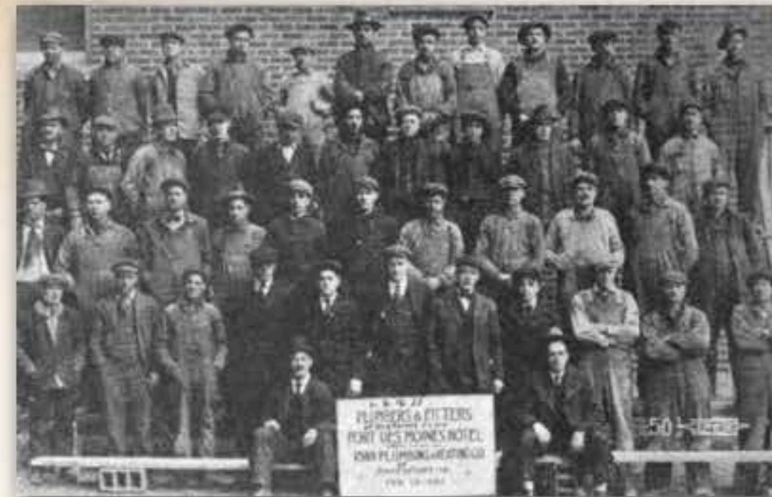
Local 33 members working for Ryan Plumbing and Heating on construction of Fort Des Moines Hotel in 1918 and 1919 included (left to right, starting at top) A. Burnside; George Hunt; Paul Pennington, assistant superintendent of heating; William Robinson; L. Feezer; Ed Spitznagle; W. Wittkowsky; W. A. Rupkey; Brother McAniff; C. J. Olson; S. L. Whitmore; George Kennedy; P. A. Kehoe; S. A. Moran; Martin McGlone; Joe Fox; Charles Miller; Jerry Brown; Victor Merchant; Steve Crary; George Gerber; Harry Loring; Oscar Sparland; Tom Lynch; C. W. Stall; Charles Arkill; Charles Crary; H. E. Korneman; Joe Kohler; Dan Baldwin; William Ammison; C. Otto; Joe Burkehead; Robert Gilmore; W. E. Bunton; Dave Morgan; Paul Gustafson; W. C. Shanley; Roy Wiseman, superintendent of heating; Patrick Mansfield, superintendent of plumbing; M. Sandler, timekeeper; A. Isbell; W. E. Dike; Robert Haslett; Frank Wilson, assistant superintendent of plumbing; and J. W. Conklin, business agent.
